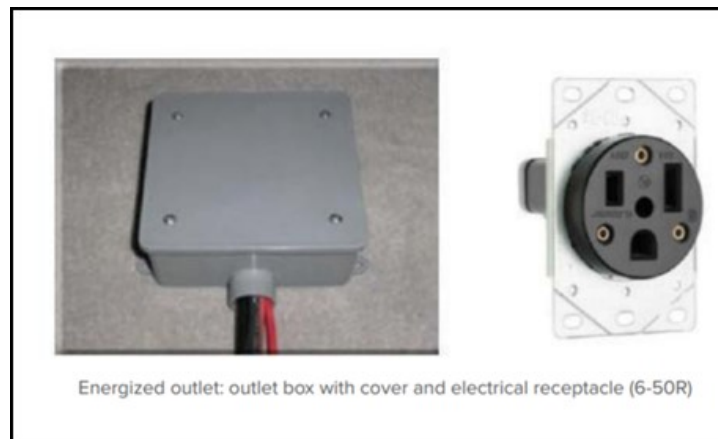
Figure 8 An energized outlet, intended for the eventual installation of a Level 2 electric vehicle charging station (240V)
