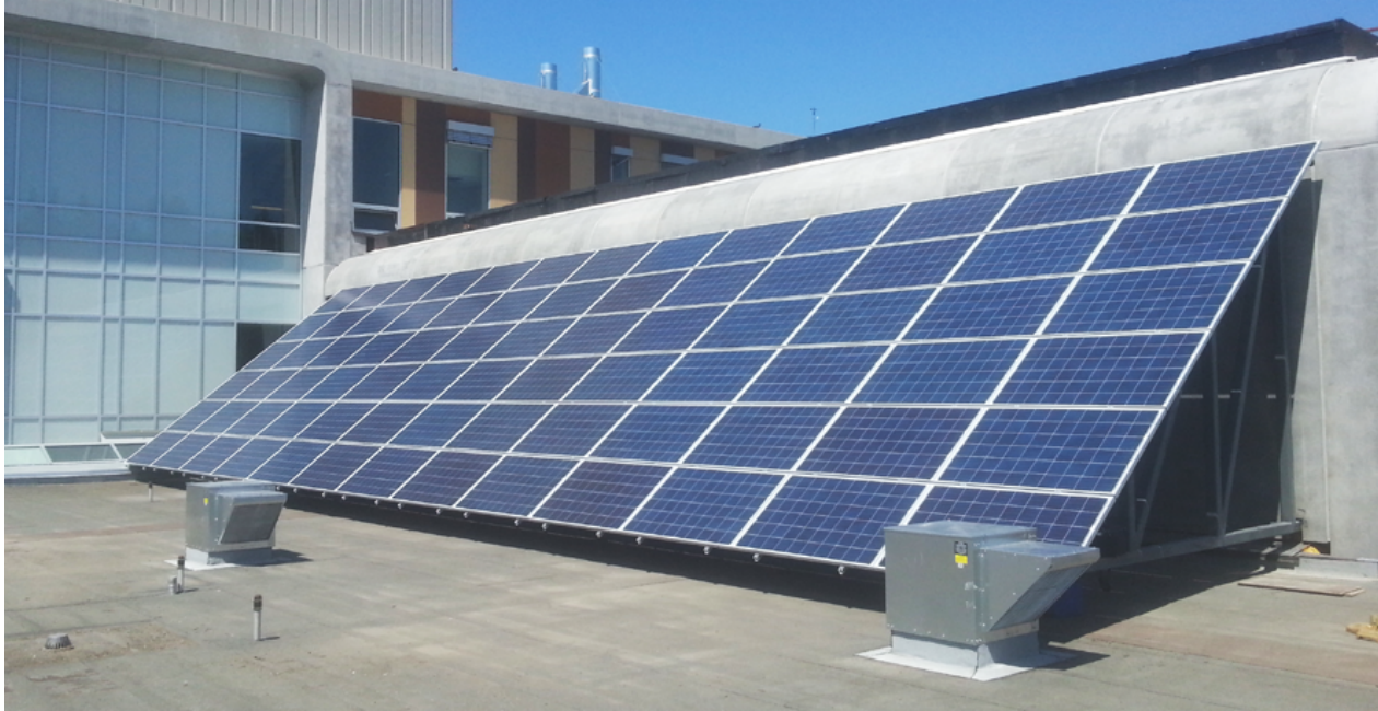
20 kilowatt solar photovoltaic grid-tie panels, St. Mary's Hospital
